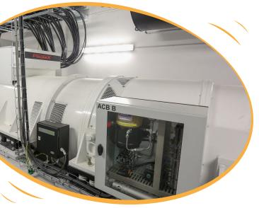
In the case of a power outage, supercomputers and their support technology are powered by an emergency backup diesel generator. This temporary power source can supply energy to Salomon and the entire IT4Innovations building for about 60 hours.
